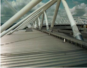
GRP Grating is an excellent choice for Rooftop walkways – they are light weight compared to metal, offer high strength, excellent non slip properties in any kind of weather, UV Stable, can easily be cut on site.
