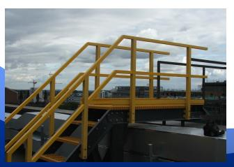
GRP Is an excellent product to use when producing a platform for a roof. GRP is extremely strong, lightweight, UV stable weather resistant.
